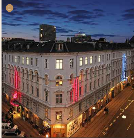
Urban House Copenhagen by MEININGER 228 rooms
